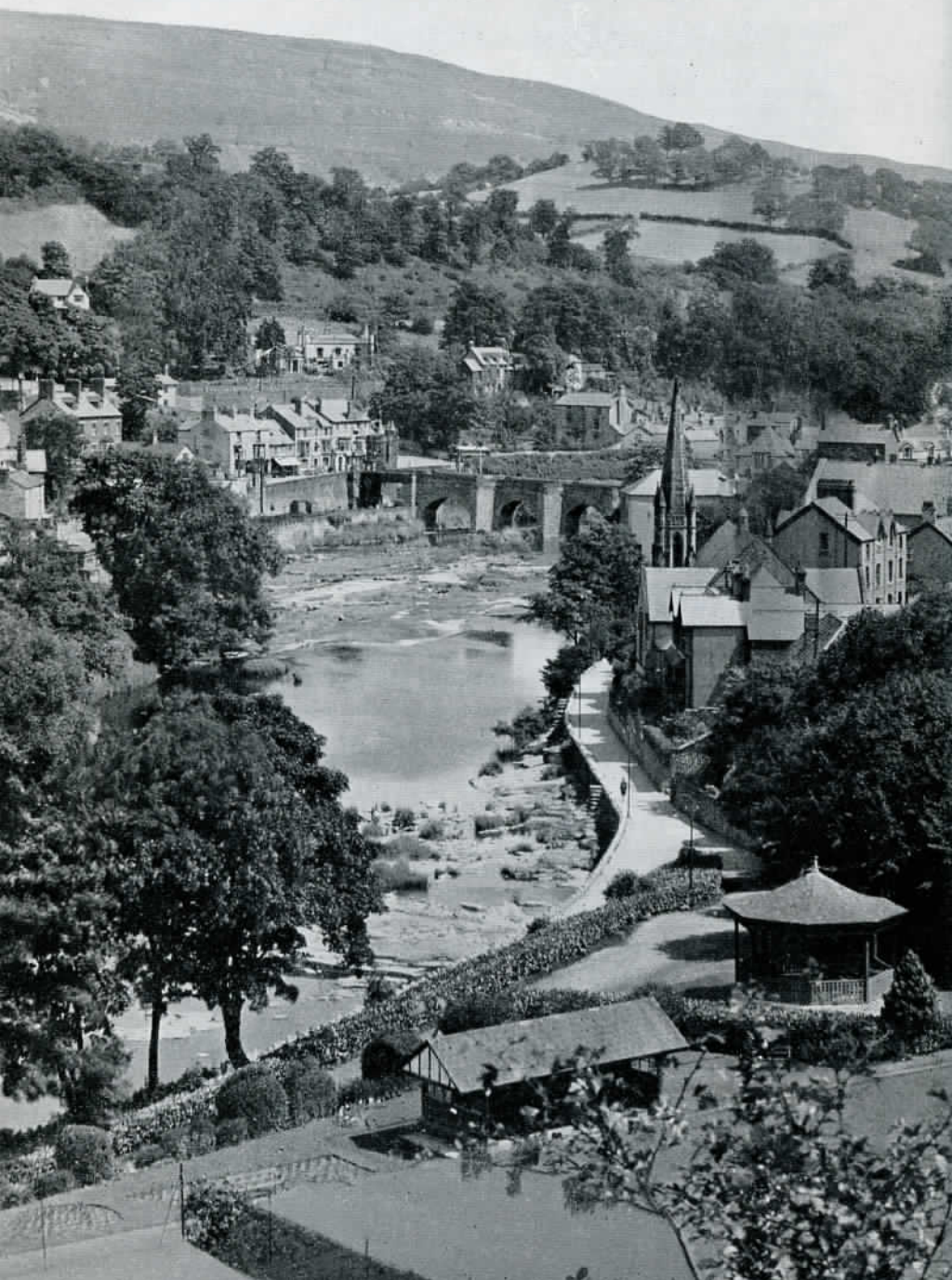
VIEW FROM RIVERSIDE PARK
